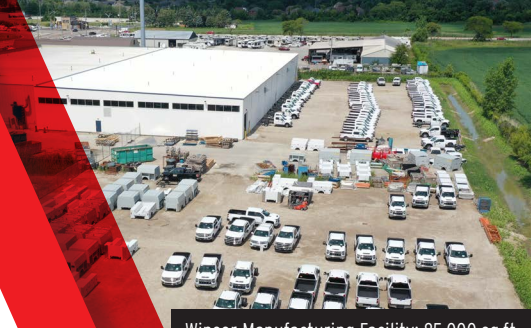
Winsor Manufacturing Facility: 85,000 sq.ft
